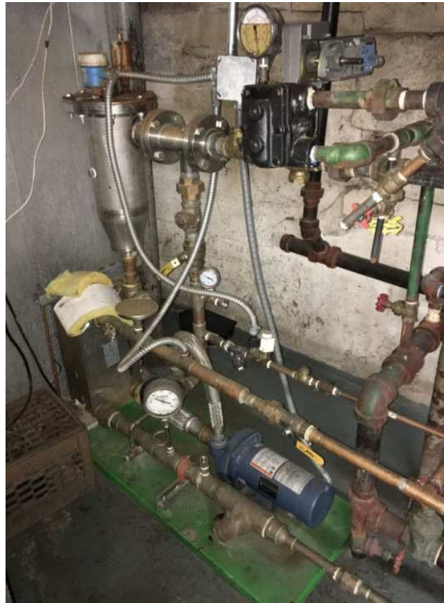
Figure 6. Fisonic Device, Vortex Tank, Plate and Frame Heat Exchanger and Water Pump.
